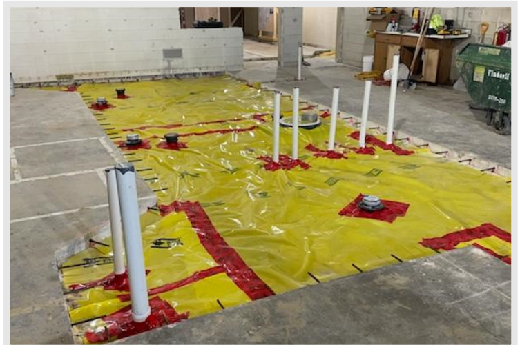
Findorff labor crews working to prepare concrete slab in-fills for pourback. Findorff concrete crews will pour these in-fills in the coming days.
